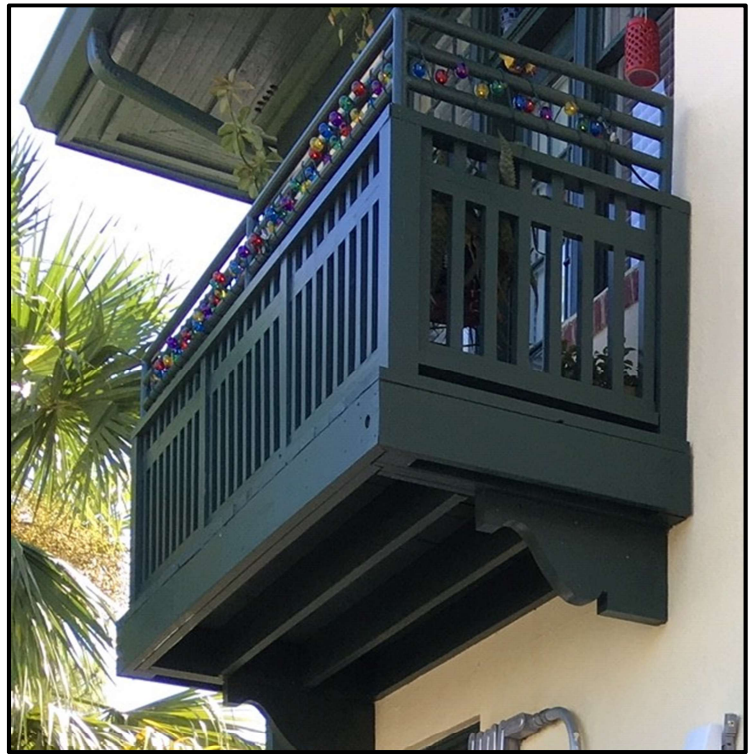
Rebuilt balconies to code height
